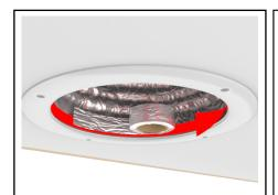
Attach flexi shaft to inside of ceiling ring collar with aluminium tape provided.
